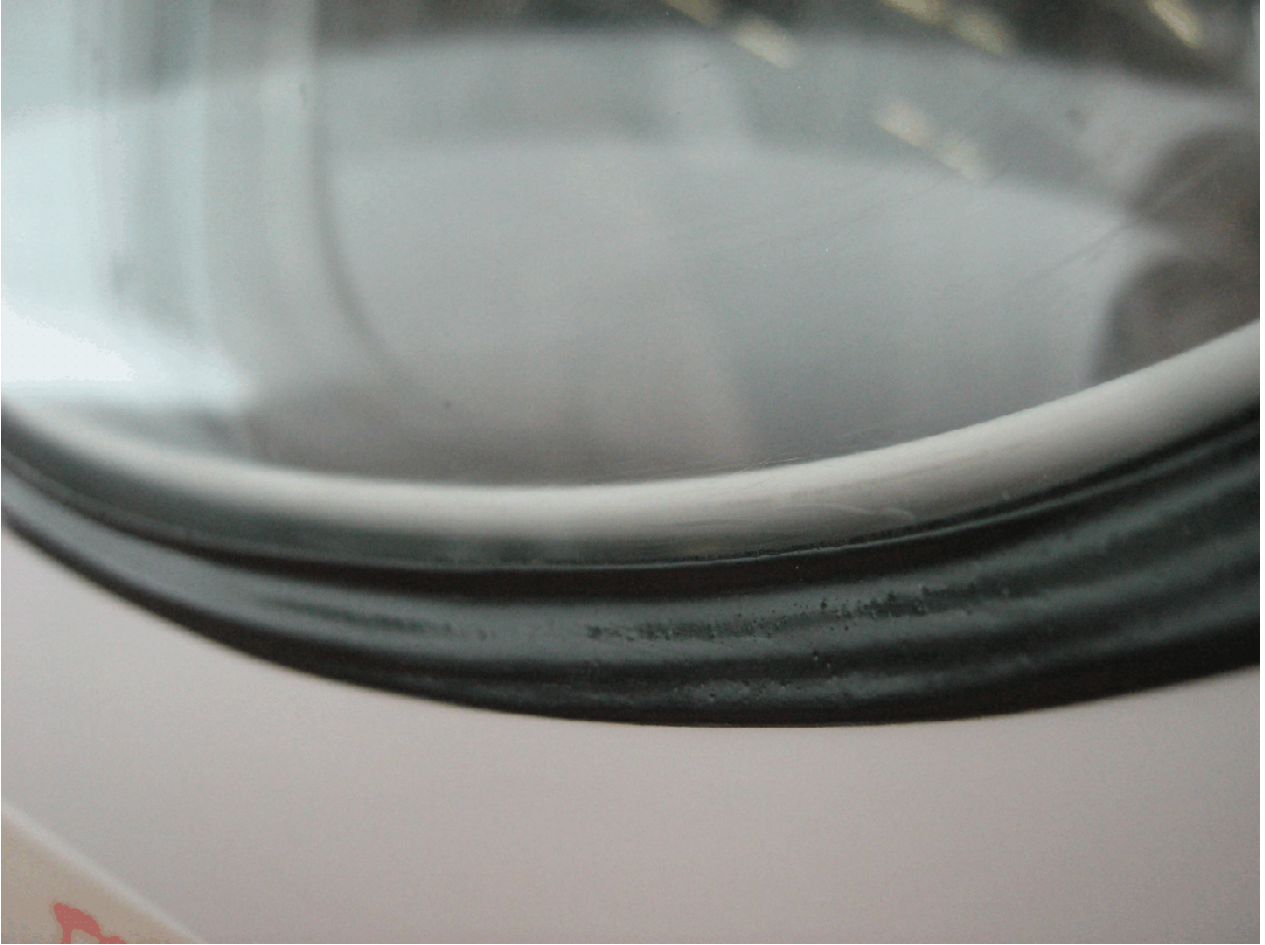
Fig. 205 - Cabin Window External Sealant - Restore (Sheet 4 of 4)
