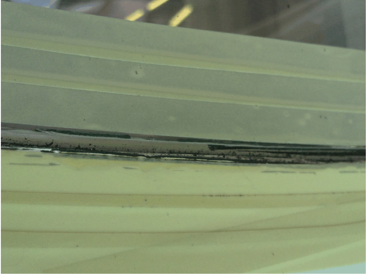
Fig. 205 - Cabin Window External Sealant - Restore (Sheet 2 of 4)
